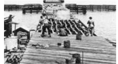
Building Wooden Bridge
