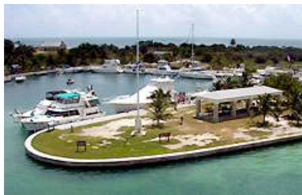
HYC on the Boca Chita wall
